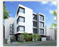
Completed in Mar 2013
