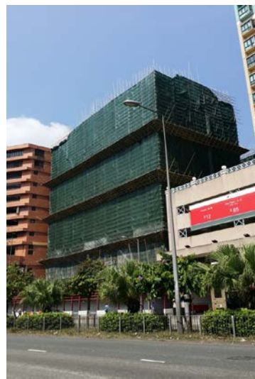
Original building while undergoing demolition
