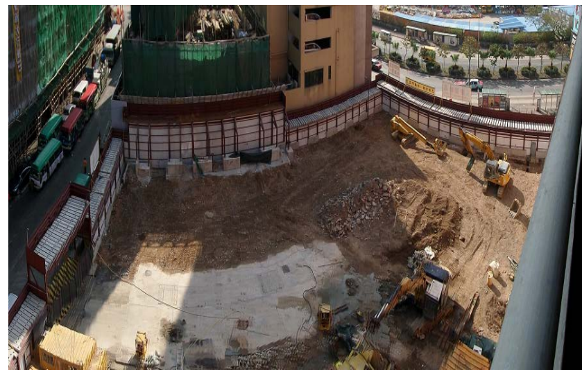
Current land after demolition
