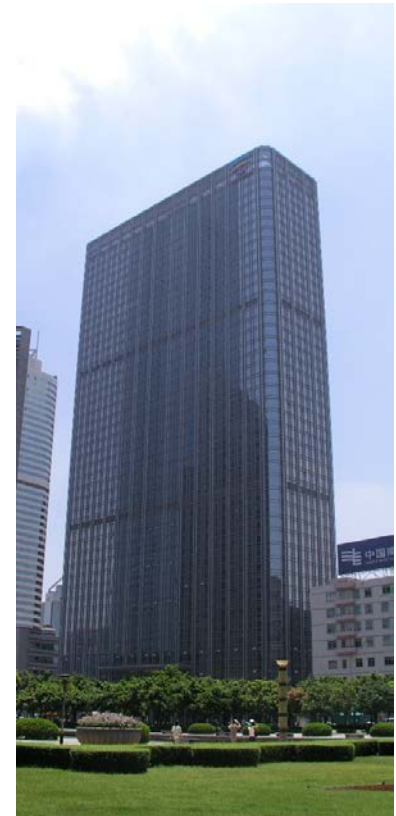
China Shine Plaza in Guangzhou, China
