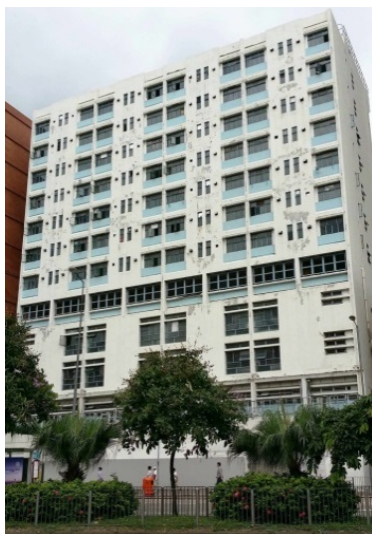
Original building on the land before demolition
