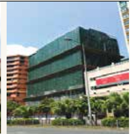
2. Original building while undergoing demolition
