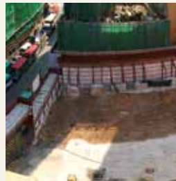
3. Current land after demolition
