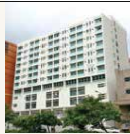
1. Original building on the land before demolition
