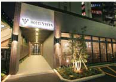
Hotel: Hotel Vista Ebina Location: Ebina, Kanagawa Number of rooms: 176
