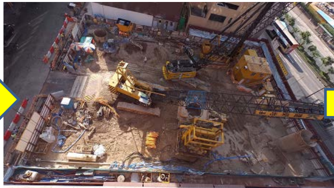
Site after demolition undergoing foundation work
