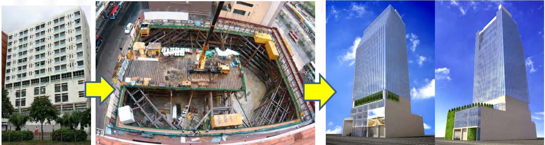
Original building on the land before demolition
