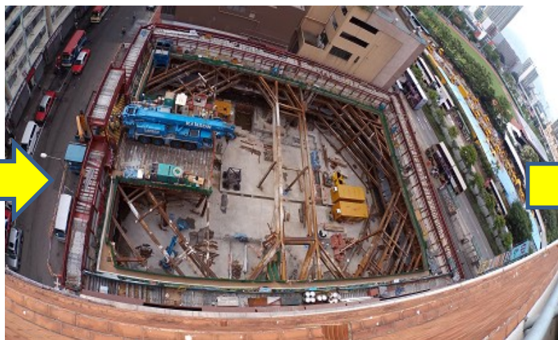
Site under construction
