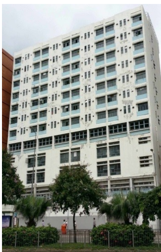
Original building on the land before demolition
