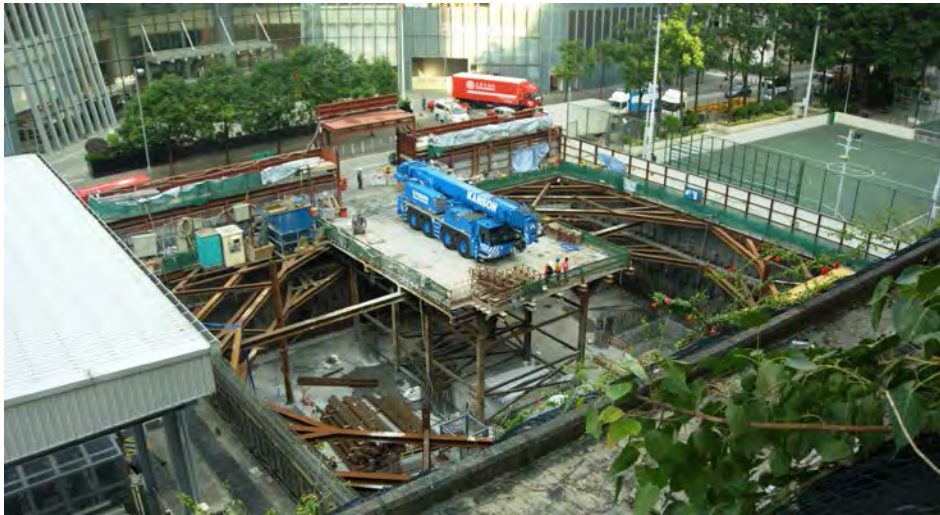
Existing site undergoing construction
